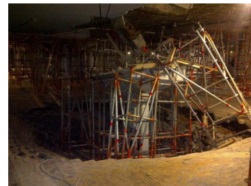
Structure after collapse
